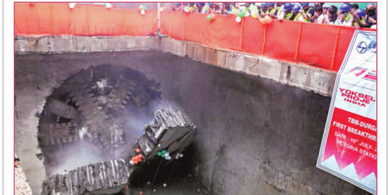
Tunnel breakthrough ceremony of the first Tunnel Boring Machine (TBM), named Durga, at the under-construction Victoria Metro station on the Khidderpore-Victoria section of the Kolkata Metro, in Kolkata, on Friday
